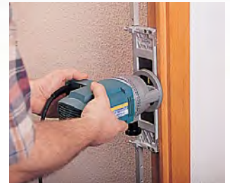
Fitting hinges with the CPN66 head.
